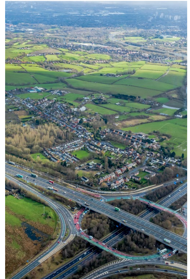
Figure 44: Aerial view of Junction 18 and Simister Lane
